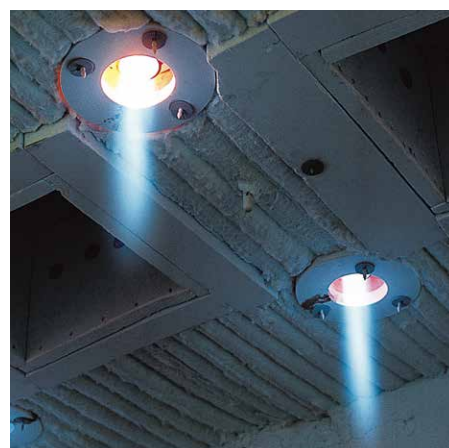
Overhead firing with BIC burners
