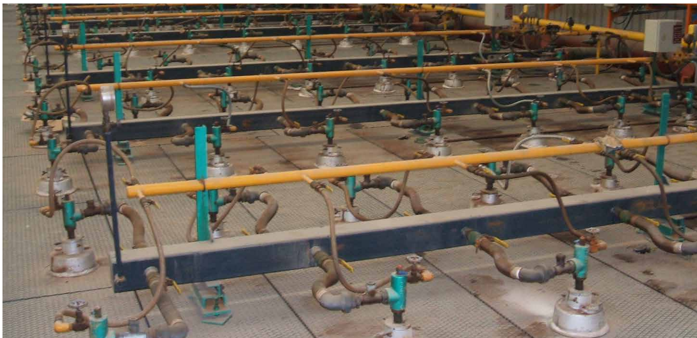
Extenso-Heat lance burners installed on the rooftop of a ceramics tunnel kiln
